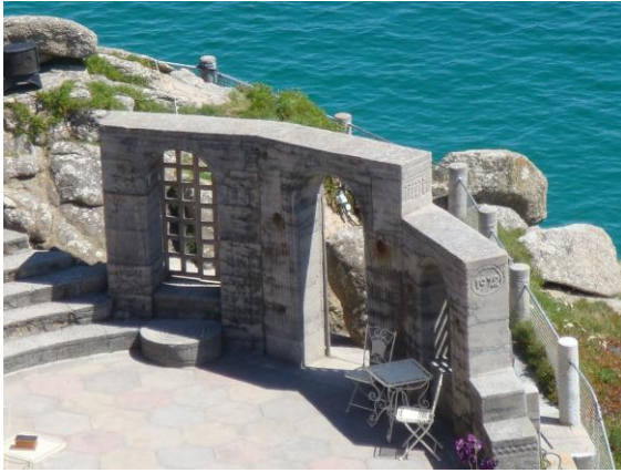
Minack Theater in Penzance
